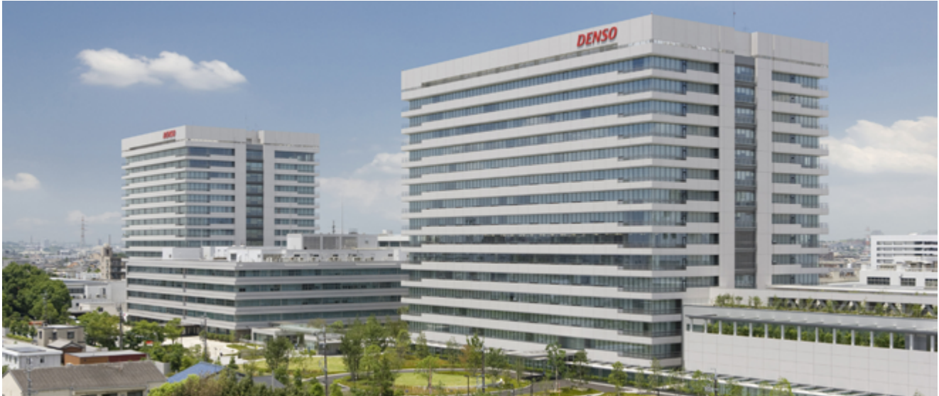
FIG. 1 DNITS provides IT infrastructures including a private cloud environment for DENSO Corporation and its subsidiaries (DENSO).
